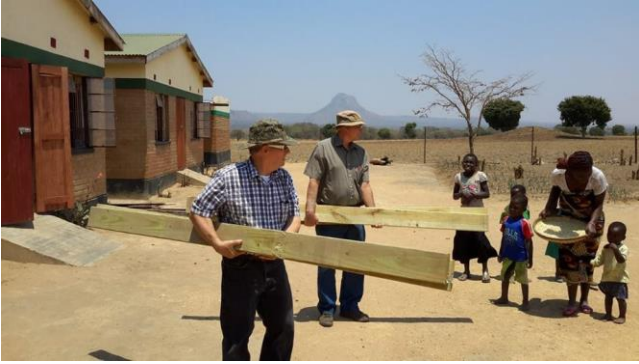
Working on installing the swing set Rev. Don Postell and Rev. David Shows.
